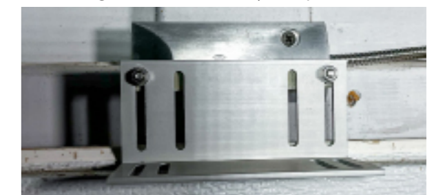
Magnet installed using optional bracket
