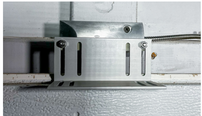
Magnet installed using optional bracket
