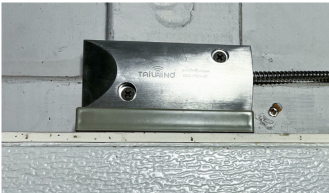
Magnet attached directly to top of door
